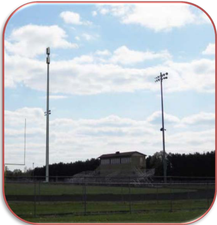
Example of “stealth” telecommunication facility placement at a high school athletic field complex.
